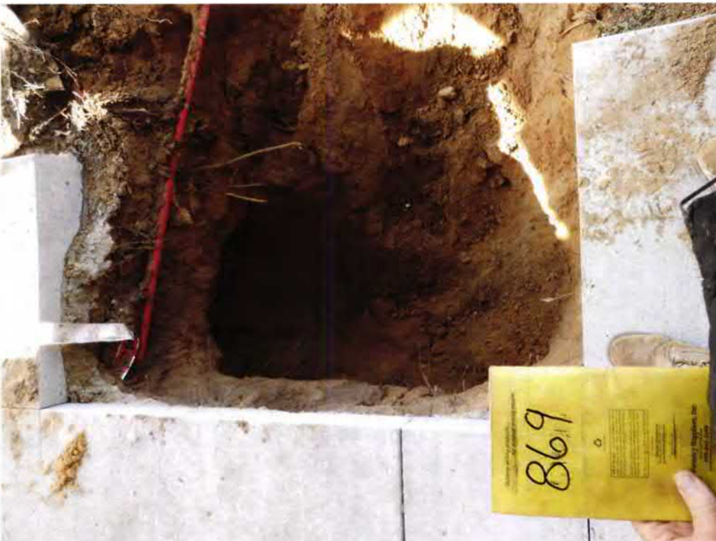
Picture 2: UST 869Cobia excavation.
